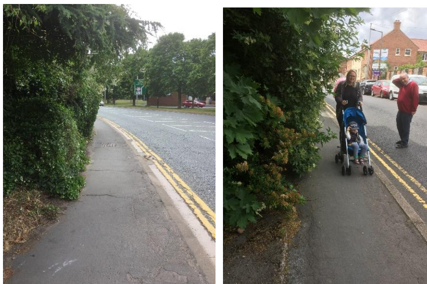
Figure 4 Pedestrian Hazards - Poor Quality Pavements
